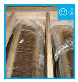
Chase is capped with rigid air barrier, duct work is sealed
