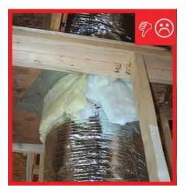
Fibrous insulation will not create air seal at duct penetration
