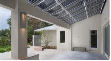
PV *IS* the roof for this back porch and covered roof-top deck.
