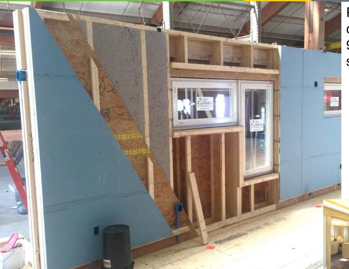
Panelized factory construction with 9.5-inch I-joist wall studs.
