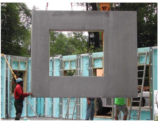
Insulated concrete panels assemble quickly on site, sit on gravel, no foundation is poured.
